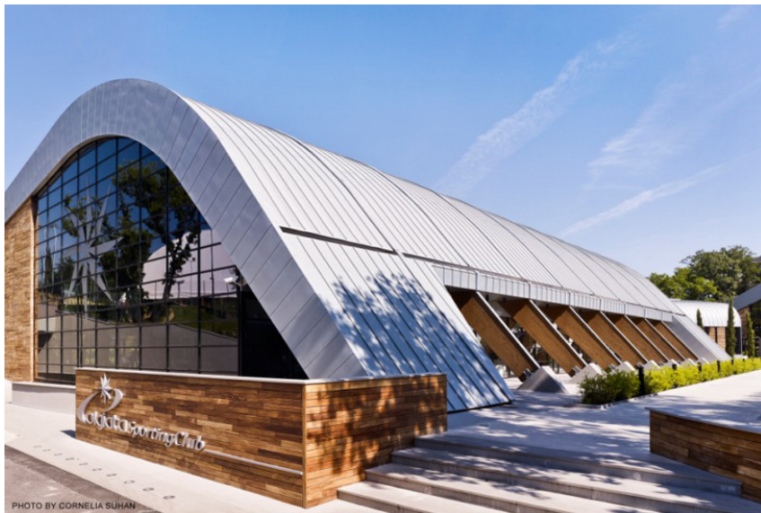
the entire roof utilizes zinc-titanium produced by rheinzink photo © cornelia suhan
