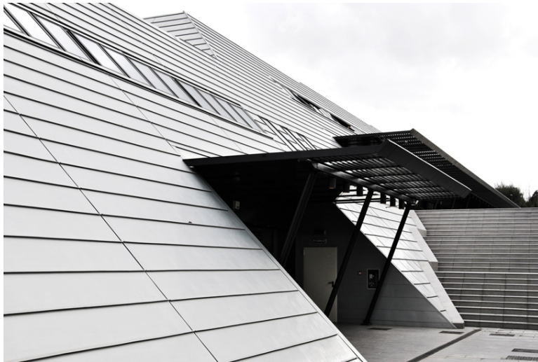
the flat-roofed structure features outward sloping sides clad in titanium-zinc
